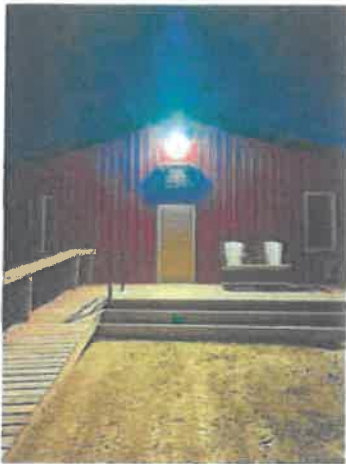
Front View of Building Showing Ramp
